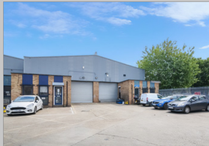
Sandgate Industrial Estate (Site 5)
