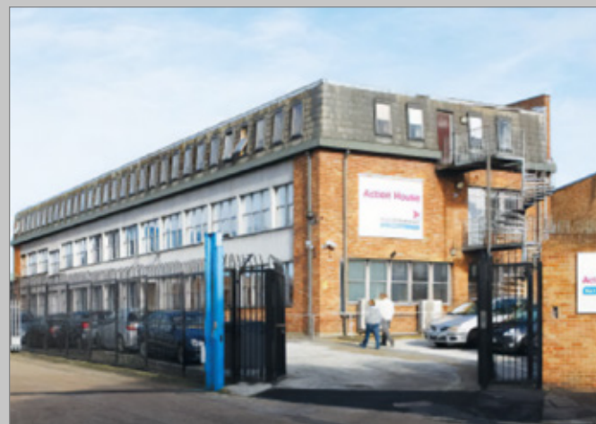
53 Sandgate Street (Site 1)
